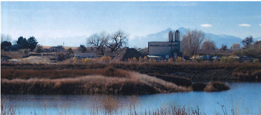
Photograph 1. Concrete batch plant, water storage pond and aggregate stockpiles.
